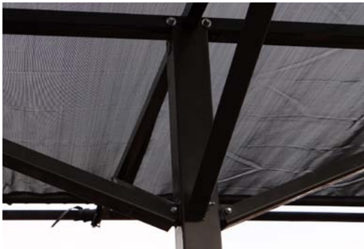
TWO 4.5" X 2.5" X 3/16" FORMED CHANNEL BRACES
