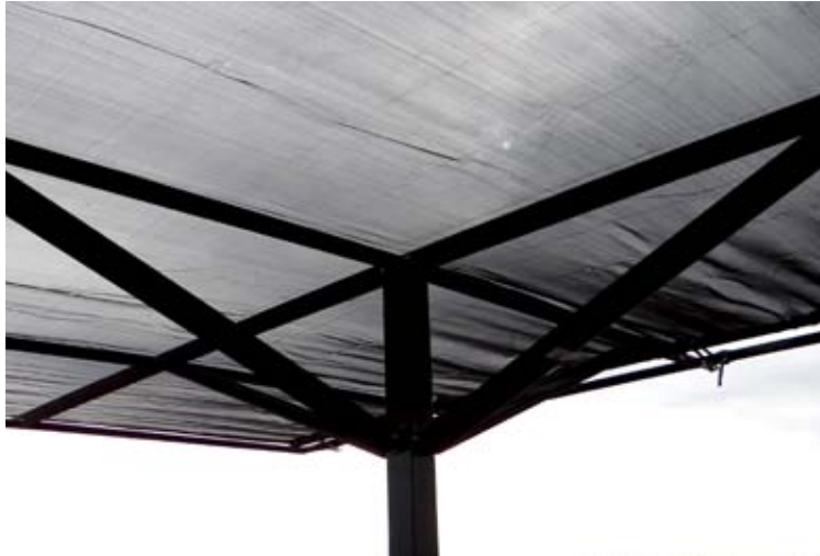
TWO 2.5" X 2.5" X 3/16" FORMED ANGLE BRACES
