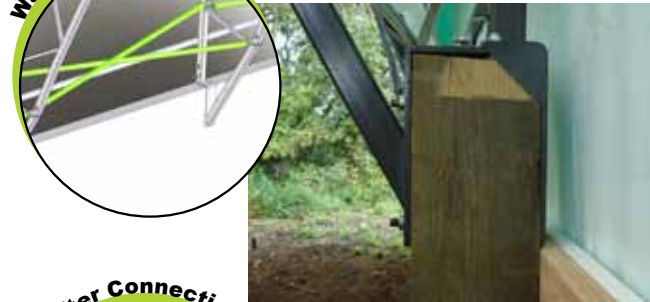
Leg To Rafter Connection
