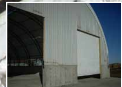
60' X 400' LIVESTOCK SHELTER Truss Legs
