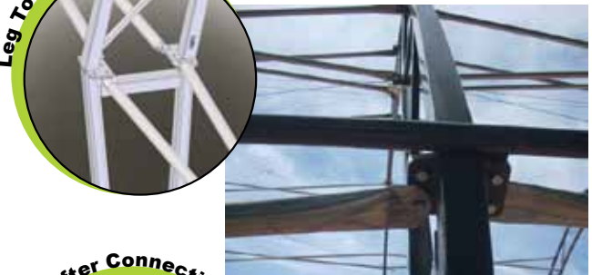
Purlin To Rafter Connection
